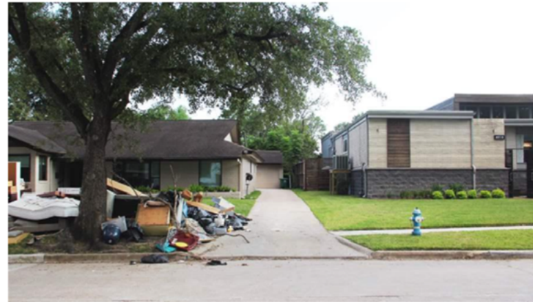
The house on the right in Meyerland, Texas, was elevated above the 100-year floodplain and largely spared damage from Hurricane Harvey while the non-elevated one on the left sustained flood damage. A new study by the National Institute of Building Sciences finds $6 saved for every dollar invested in mitigation activities to reduce risk and disaster losses.
