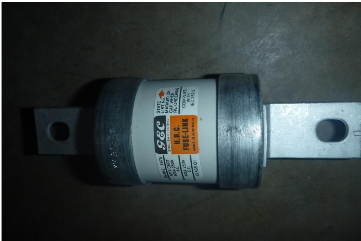
315 Amp Fuses Protecting the Output of the Generator
