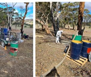
Ash Pump and Containers Vacuuming the Ash into Drums
