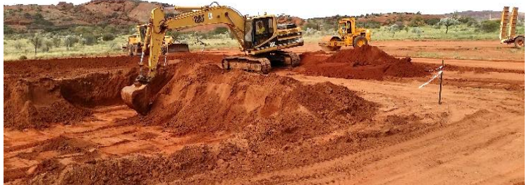
RASAC construction of earth dams (water storage) at Ronald's Bore.
